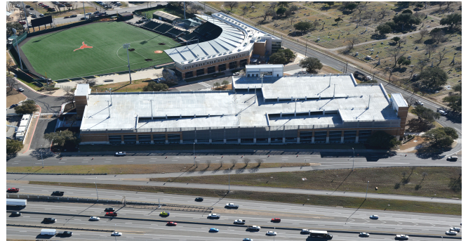
The University of Texas at Austin - East Campus Parking Garage
