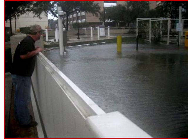
UTHSC Houston after Hurricane Ike
